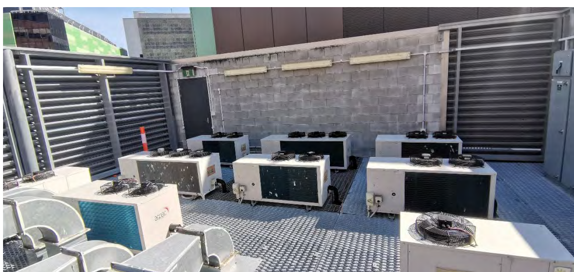
Figure 6 QCH site for Thermal-XR testing
