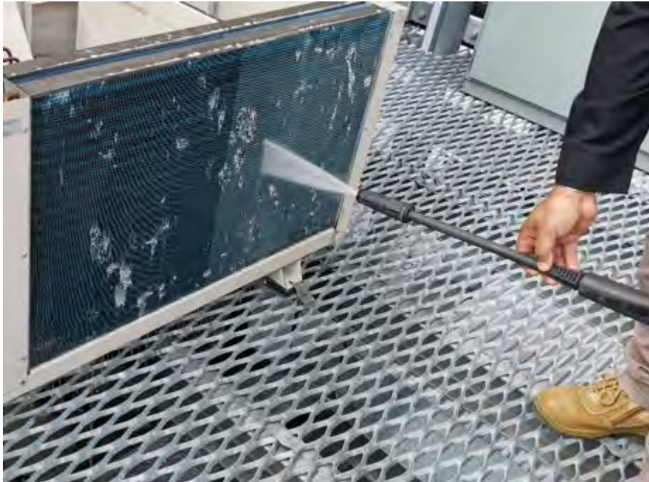
Figure 2 Cleaning process (Thermal-XR Prep)
