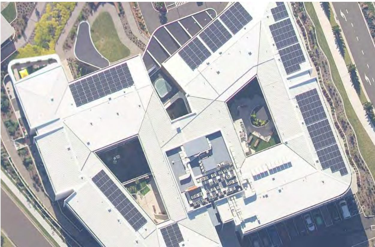
Figure 3-3 - Aerial view of the Living Laboratory with the 99 kW-p PV system and HVAC service on the roof.
