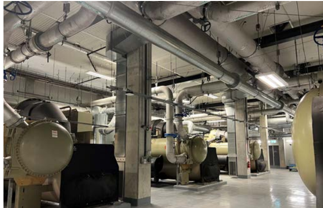
Figure 4.2 Chiller plant
