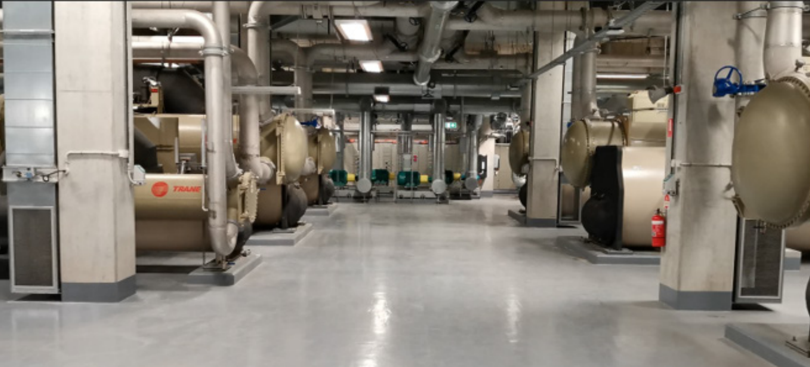
Figure 4.3 Hospital Energy plant
