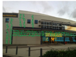
Sketch over of some of the highest scoring net zero energy design strategies including trellis and green wall, motorised louvers on the ground floor, microshade mesh in the second floor windows and BIPV/ spray on solar for the second floor glazing.
