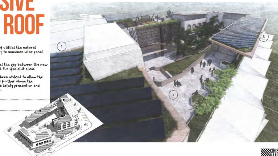
Figure 3-2 "Westcourt Living" hybrid green-solar roof – Quinlan Hatchett
