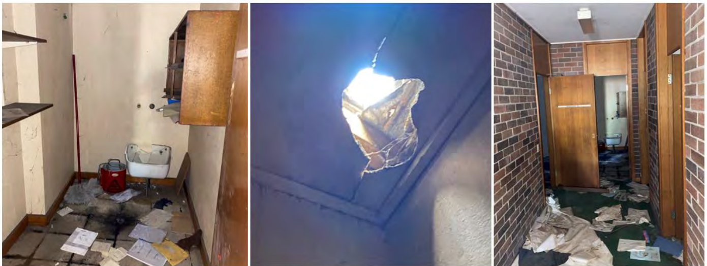
Figure 3. Current state of the former Unanderra police station site (interior)
