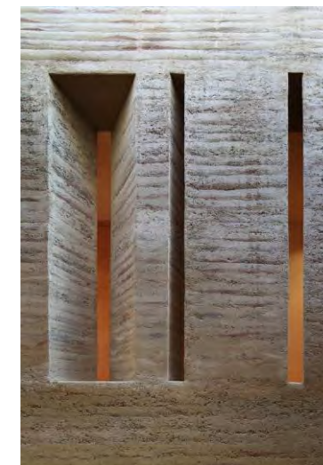
Rammed Earth is a sustainable construction material with great thermal properties https://www.wsj.com/articles/rammed-earth-luxury-homes-1427989394 (left hand image) https://www.archdaily.com/933353/how-rammed-earth-walls-are-built (right hand image)
