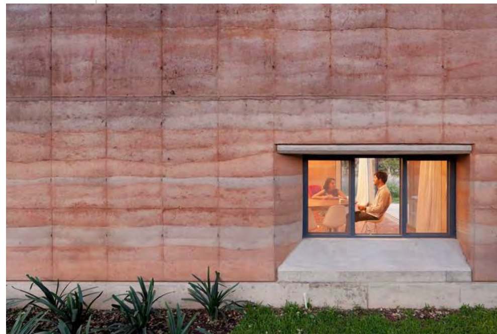
Rammed earth construction using local soil/clay with timber framed roof – low embodied carbon building materials.
