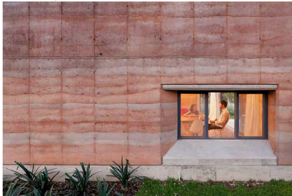
Rammed earth construction using local soil/clay with timber framed roof – low embodied carbon building materials.
