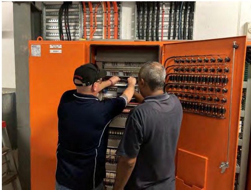
Figure 1: Installation of JACE gateway at Building Pink 9 (CDU)
