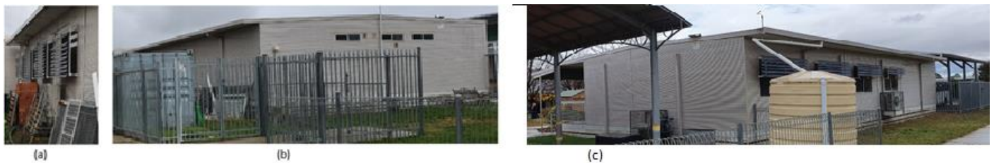
Figure 6: (a) B14 north side windows with full louvre external shading; (b) B14 north side partial low shading by shipping container, and west side high windows unshaded; B13 east side shade structure; north windows partial height shade louvres; west carport shade.
