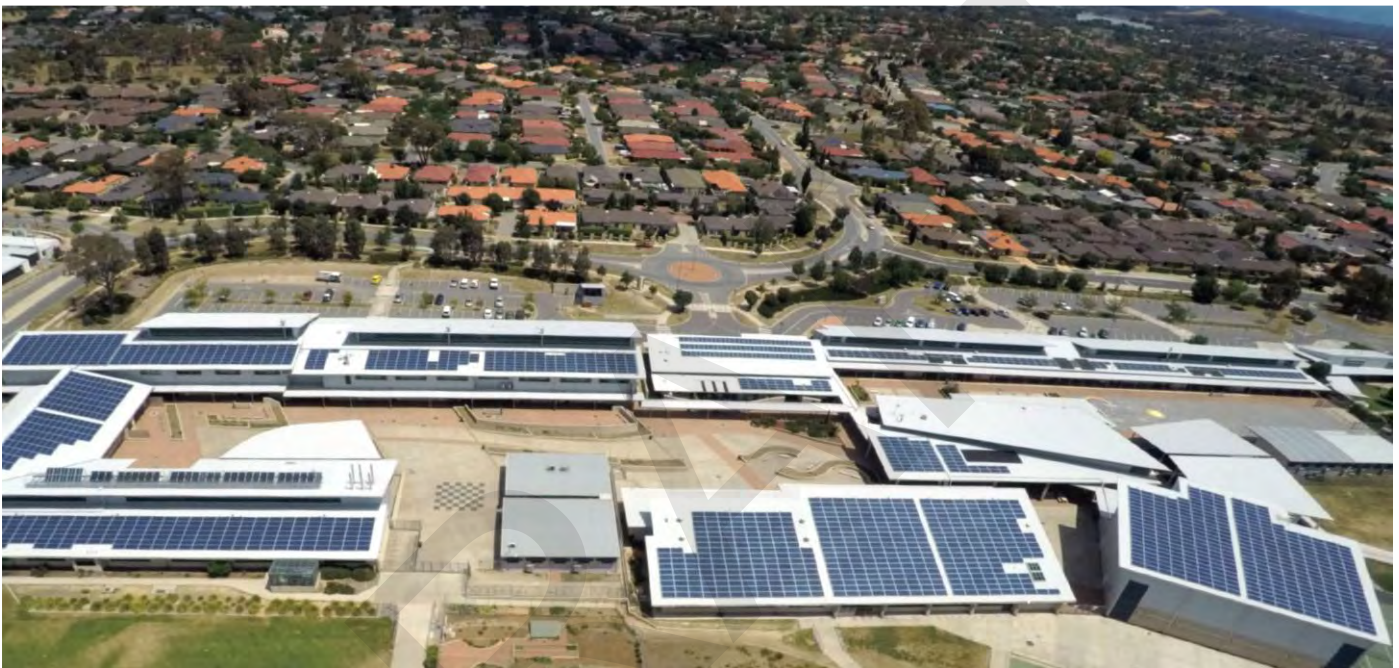
Figure 3: Amaroo School aerial view from the north featuring the 600kW solar array.
