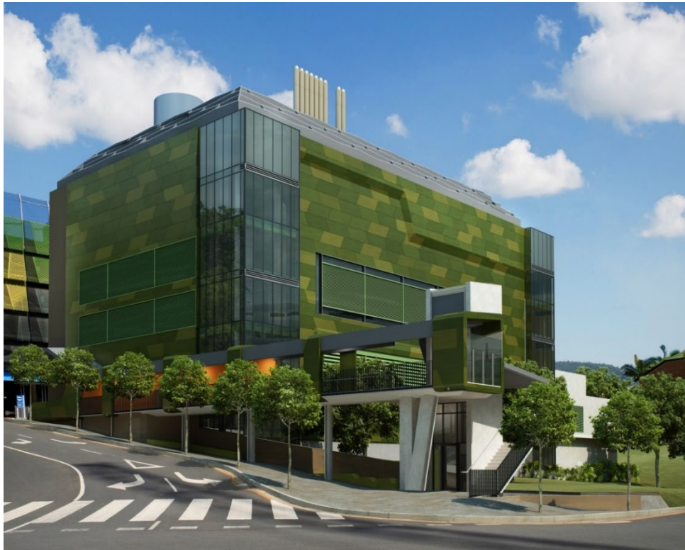
Figure 5 QCH Central Energy Plant (QCH EP) Building
