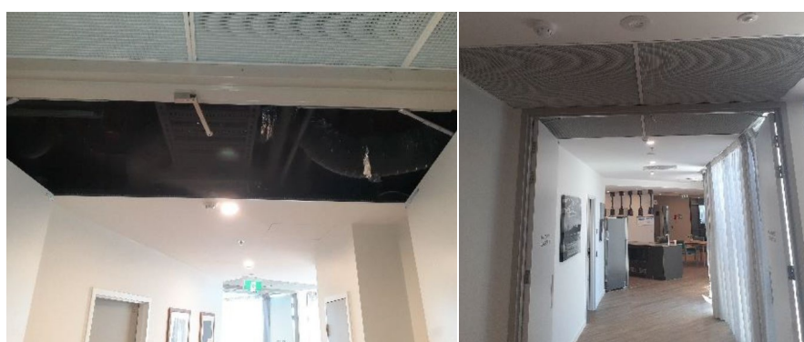
Figure 3-17 Openings in the ceiling space
