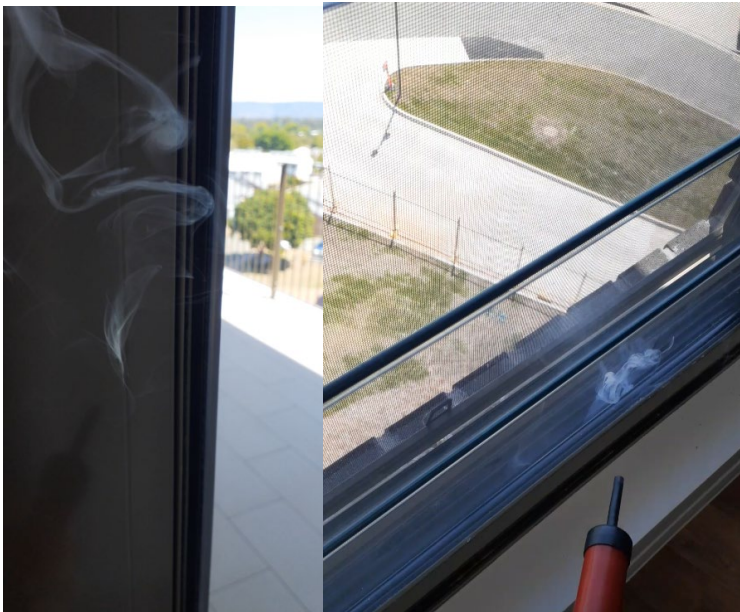
Figure 3-16 Air leakage path in windows
