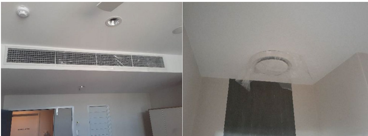
Figure 3-13 Sealing supply and exhaust
