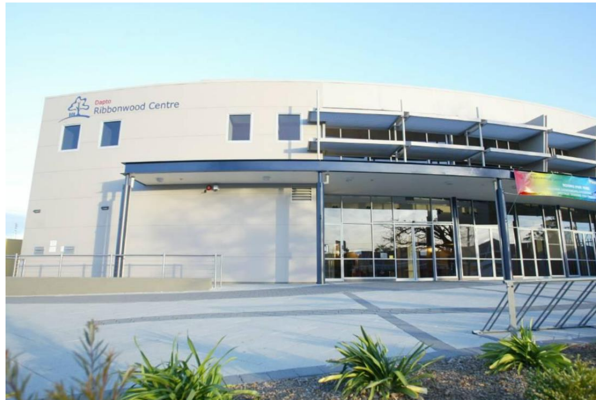
View of Entrance Atrium from Princes Highway
