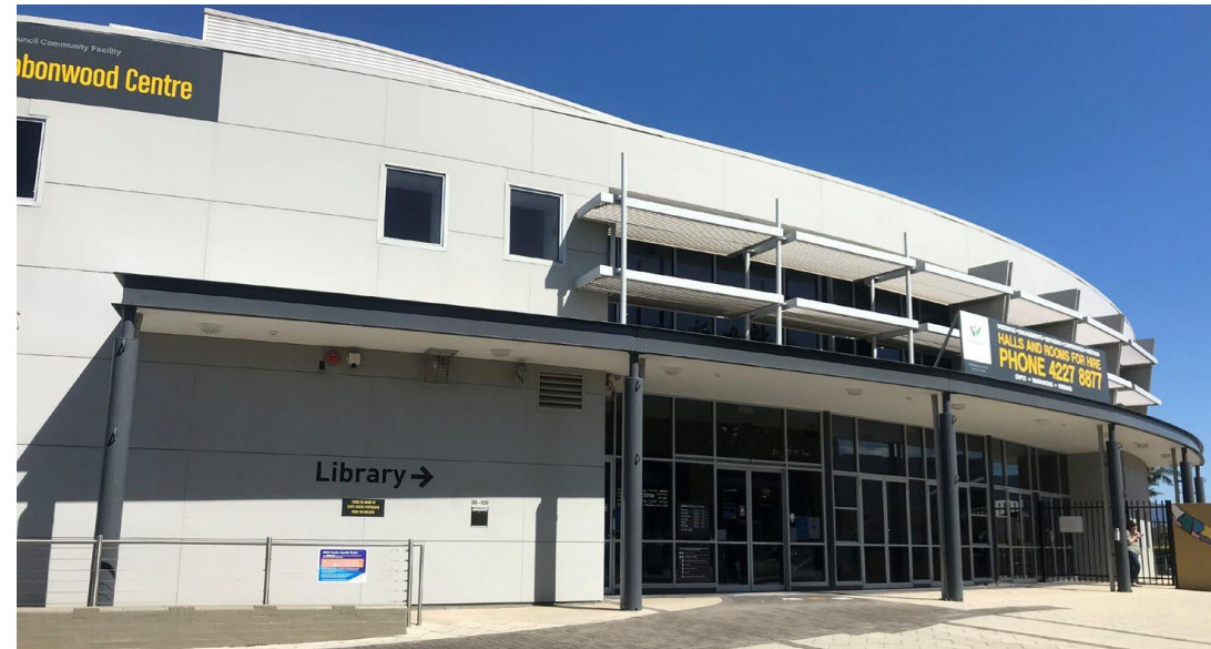
Ribbonwood Centre Entrance
