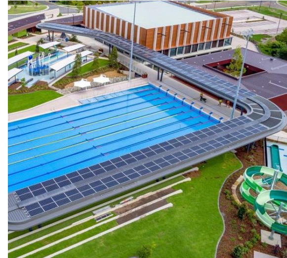
Aquatic centre electrification and extensive integration of solar PV
