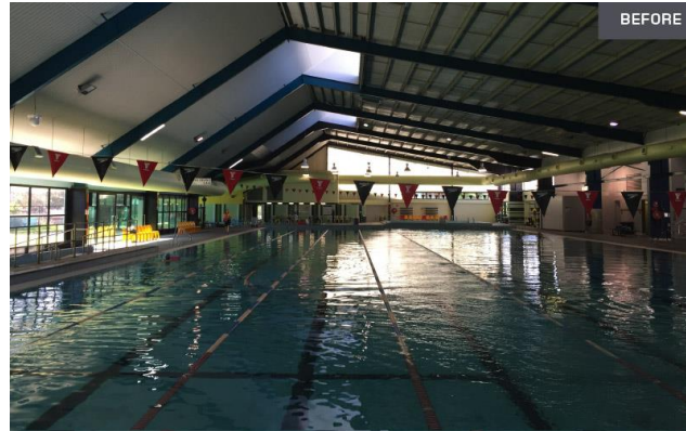
Public pool showing potential surface glare hazard
