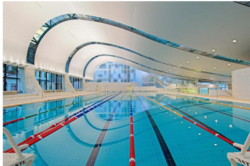
Ian Thorpe Aquatic Centre, Harry Seidler - Finishes and form used to control light quality and noise quality
