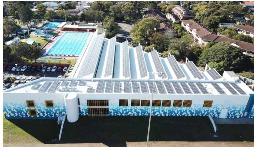
Manly Aquatic Centre retrofit showing saturation with solar PV
