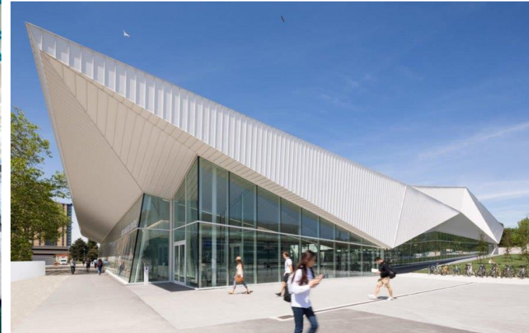
UBC aquatic centre by Ostroy Architects, Vancouver. Showing roof structure used to provide shading and to moderate the extent of façade glazing
