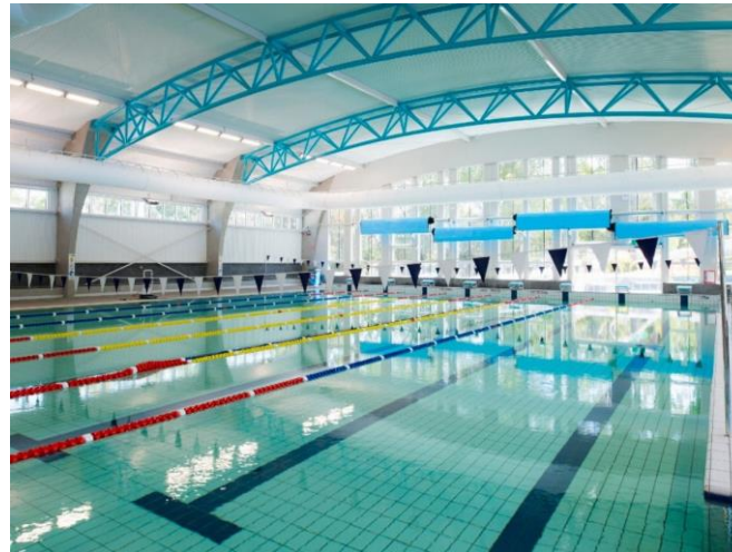
UTS Sydney by DCM, 6 Star Green Star showing one large glazed wall but also rationalised slivers of glazing on slivers of glazing on other facades
