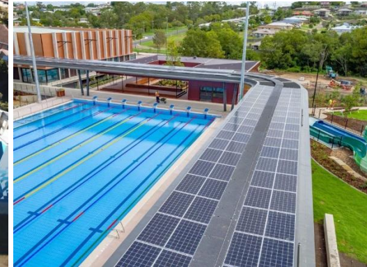
Example of solar built into shade structures around an outdoor pool
