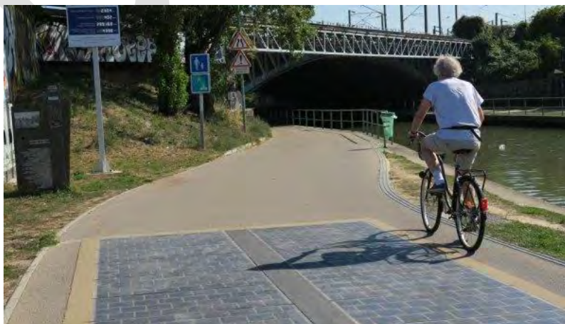
Figure 2: Wattway Road solar panels installed in Bobigny, France. Source: Wattway Website
