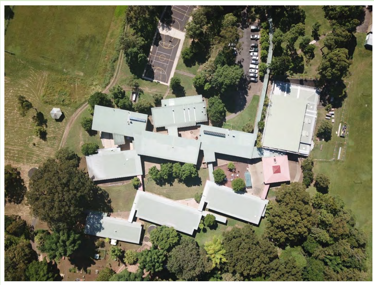
Figure 18 – Nimbin Central School – Aerial Photograph Taken During Site Visit
